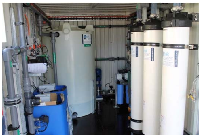
Self-contained equipment with protection from the harsh environment and including safety shower and eyewash station
