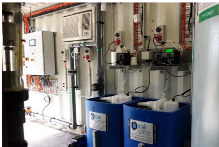
Custom design and manufacture of a 165 m 3 /day containerised Ultrafiltration (UF) plant
